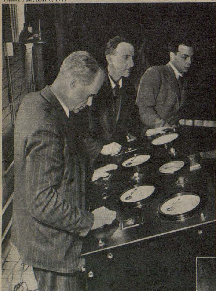
HIGH VOLTAGE TESTS: Control Desk An object is going under test at Queen Mary College Laboratory, London. In the observation gallery the operator controls the voltage.
