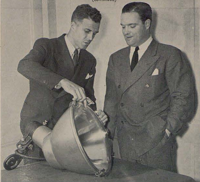
One of the 836 big lamps installed at the Polo Grounds is demonstrated by Engineer Harry Hayes of Westinghouse Electric to Horace C. Stoneham, president of the New York Giants. Lights are so designed and mounted that no player casts a shadow.
