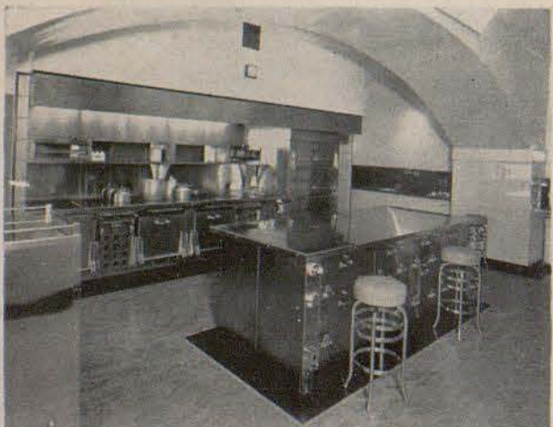
MODERNIZED KITCHEN HAS ALL ELECTRICAL EQUIPMENT
