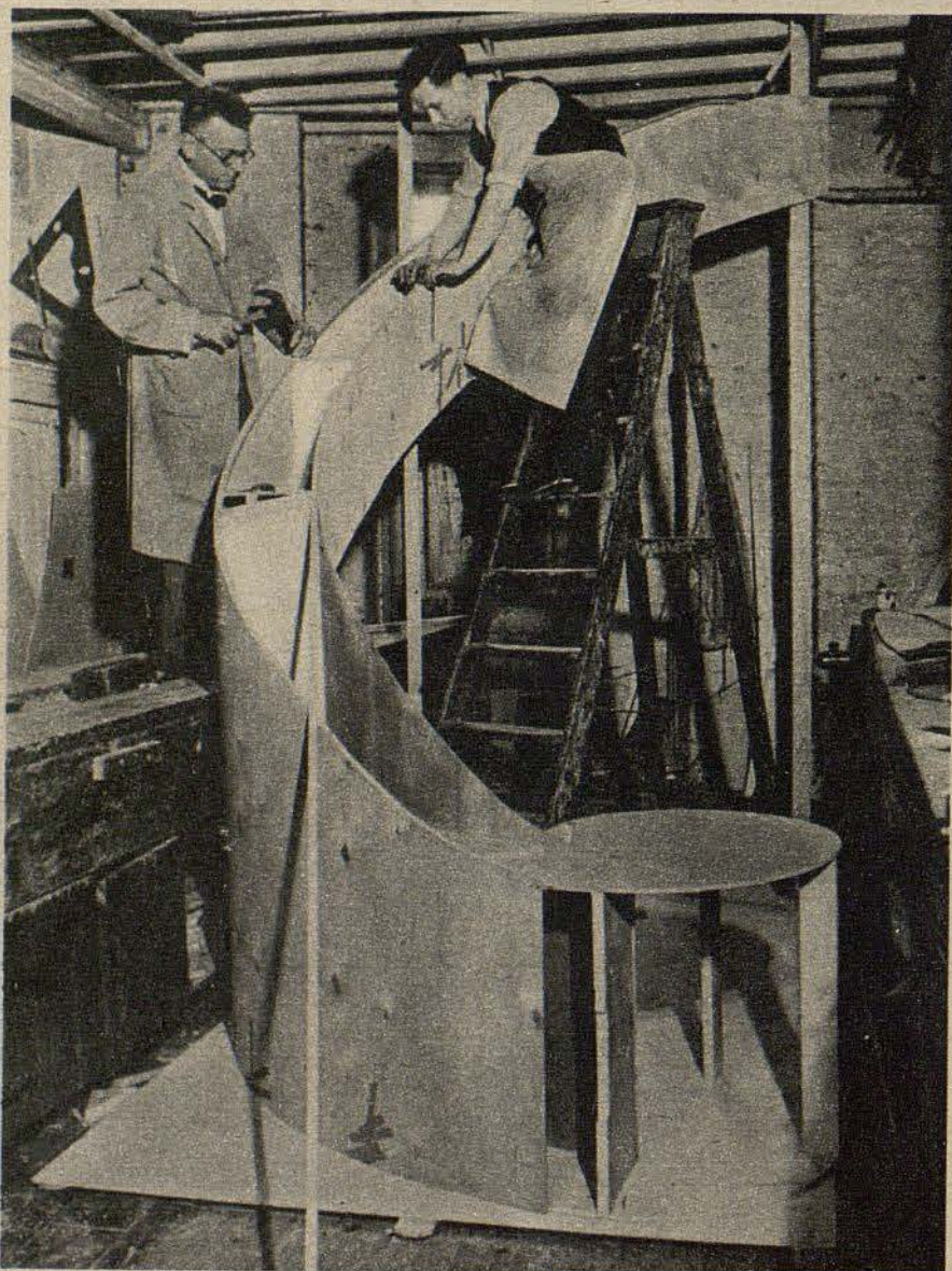
10 That marble staircase which so impresses us when we see it in the ballroom is a tribute to the art of the stage carpenter. For it is a wooden and hollow snare, but none the less palatial on that account
