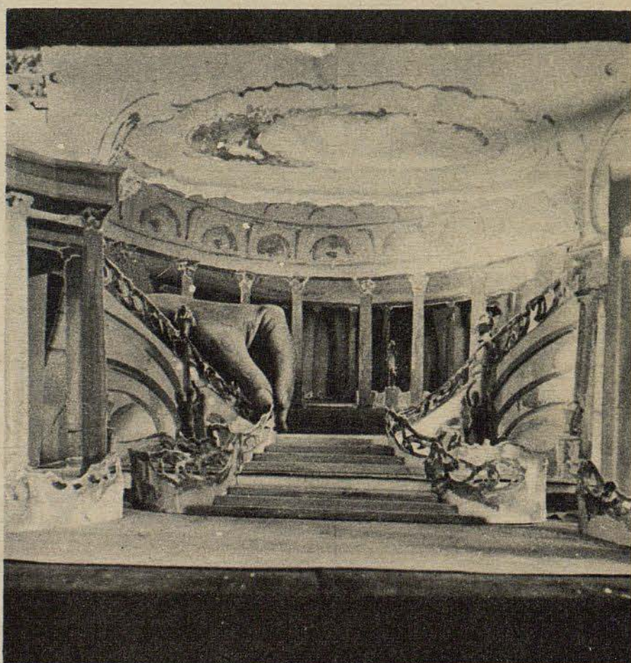
4 Before the various scenes are built in the studios, they are constructed in miniature. Hence the giant hand carefully moving a section of the elaborate banister. Use of models enables every detail to be adjusted
