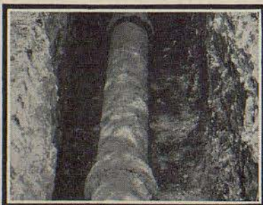
Unretouched photograph of more-than-century-old cast iron pipe still in service in Lancaster, Pa.
