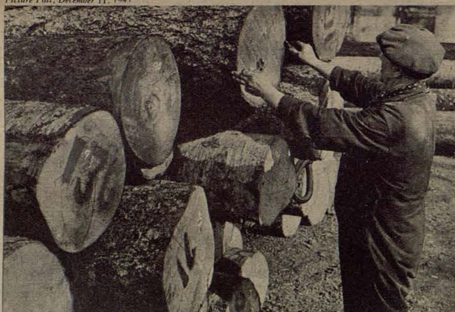
1 A LOG OF WOOD BECOMES A MOSQUITO When felled, it was given a number which will head its case history until the cutters have turned it into veneers which makes the plywood.
