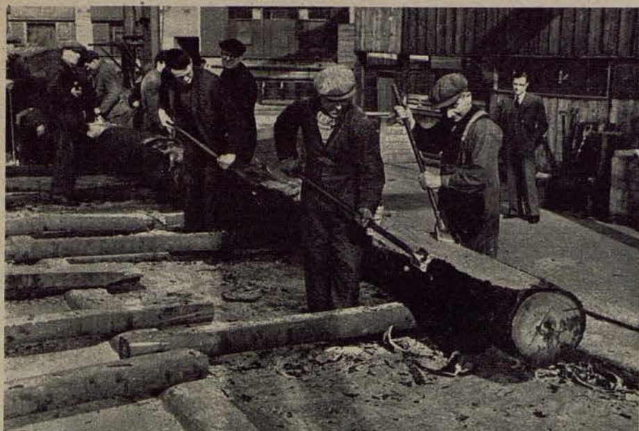
3 The Scraping that Follows the Soaking For days the logs are kept in steaming pits in order to soften them. Then the bark is taken off with huge scalpels.
