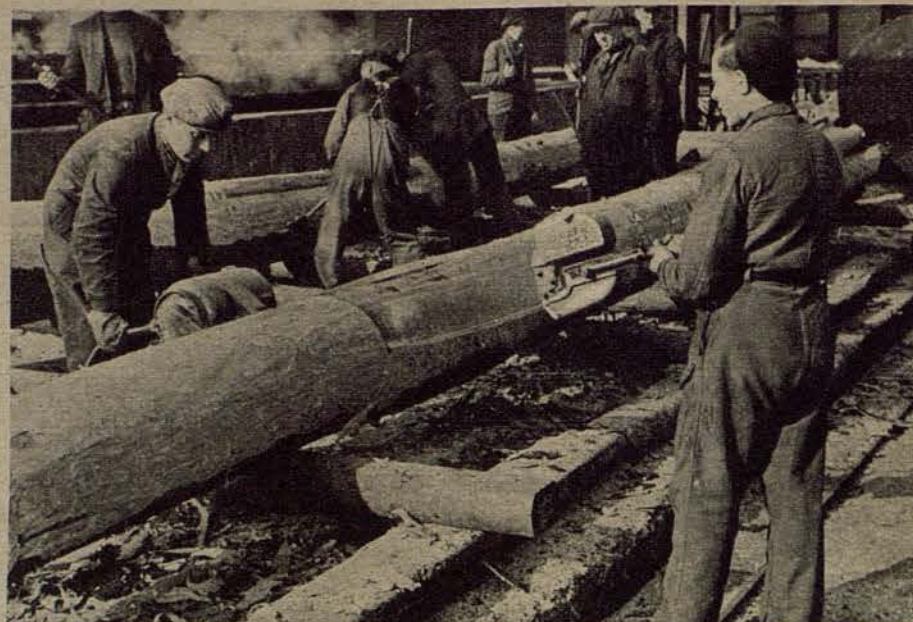
2 They Lop it into Lengths for the Peeling Machine It is cut to a length corresponding with the peeling machine's blade. The usual sizes of aircraft plywood are 5 ft. by 4 ft. or 4 ft. by 4 ft.
