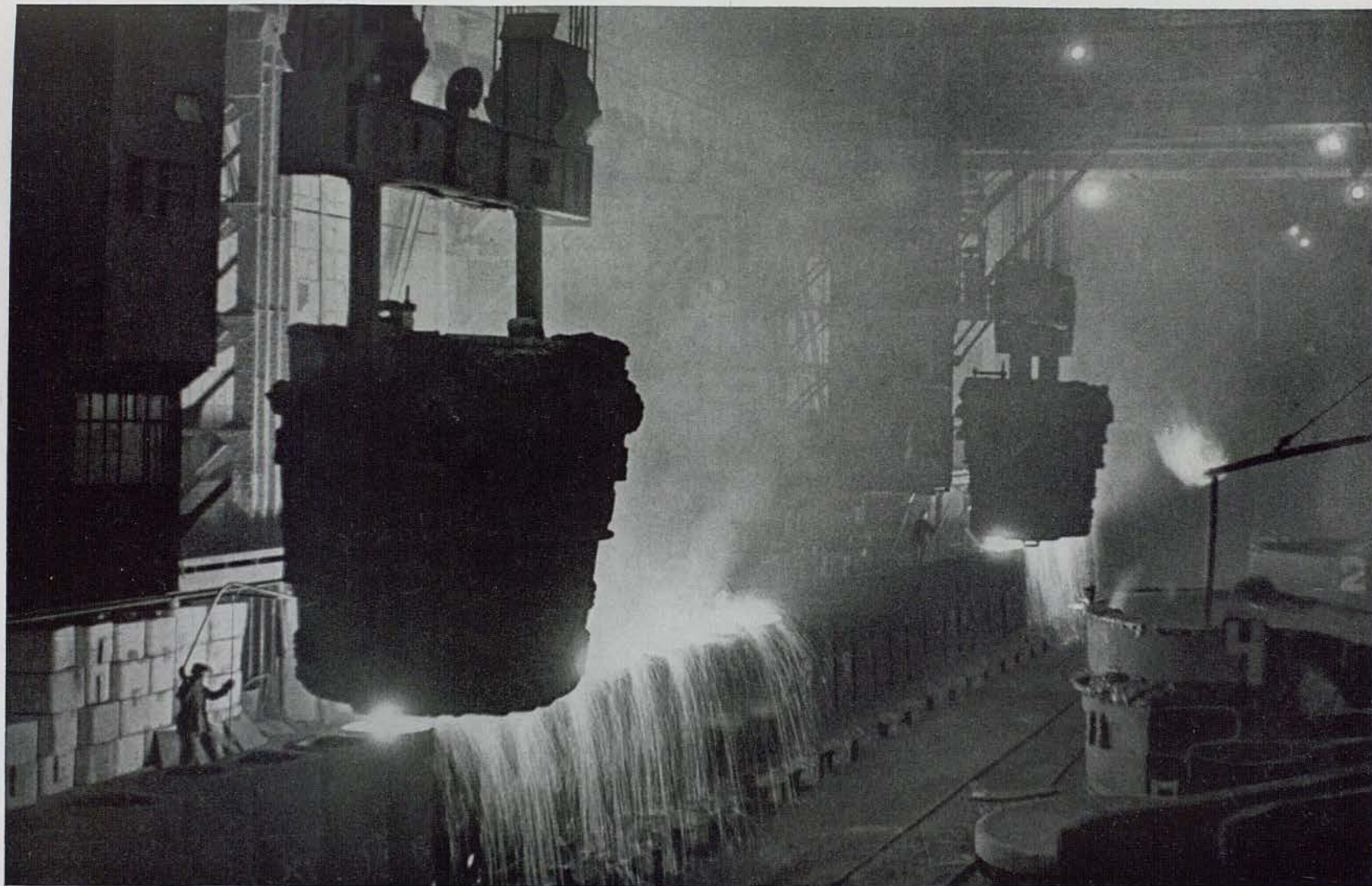
Giant Ladles, Swung from Cranes, Fill a Train of Ingot Molds with Showering White Steel from an Open Hearth at Stalinsk Dwarfing the worker, who controls its flow with a rod, the forward ladle pours molten metal through a valve in the bottom. When the last mold has been filled, the ingots will be stripped and sent to the blooming mill for rolling. Meanwhile, the open hearth, having been emptied, will receive another charge.
