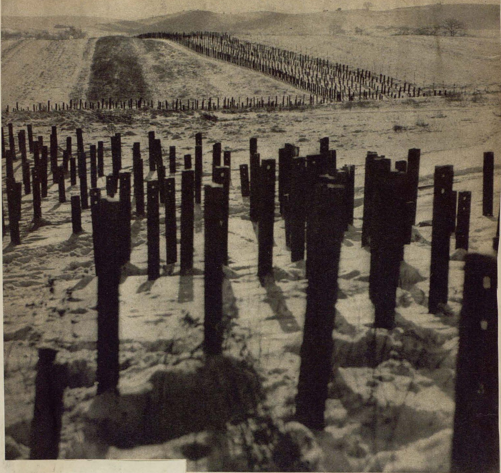
PROSPECT OF THE MAGINOT LINE : Where the Tanks Shall Not Pass The pleasant fields of Lorraine, planted with line upon line of anti-tank girders. Dim on the horizon are the turrets of yet another fortress.
