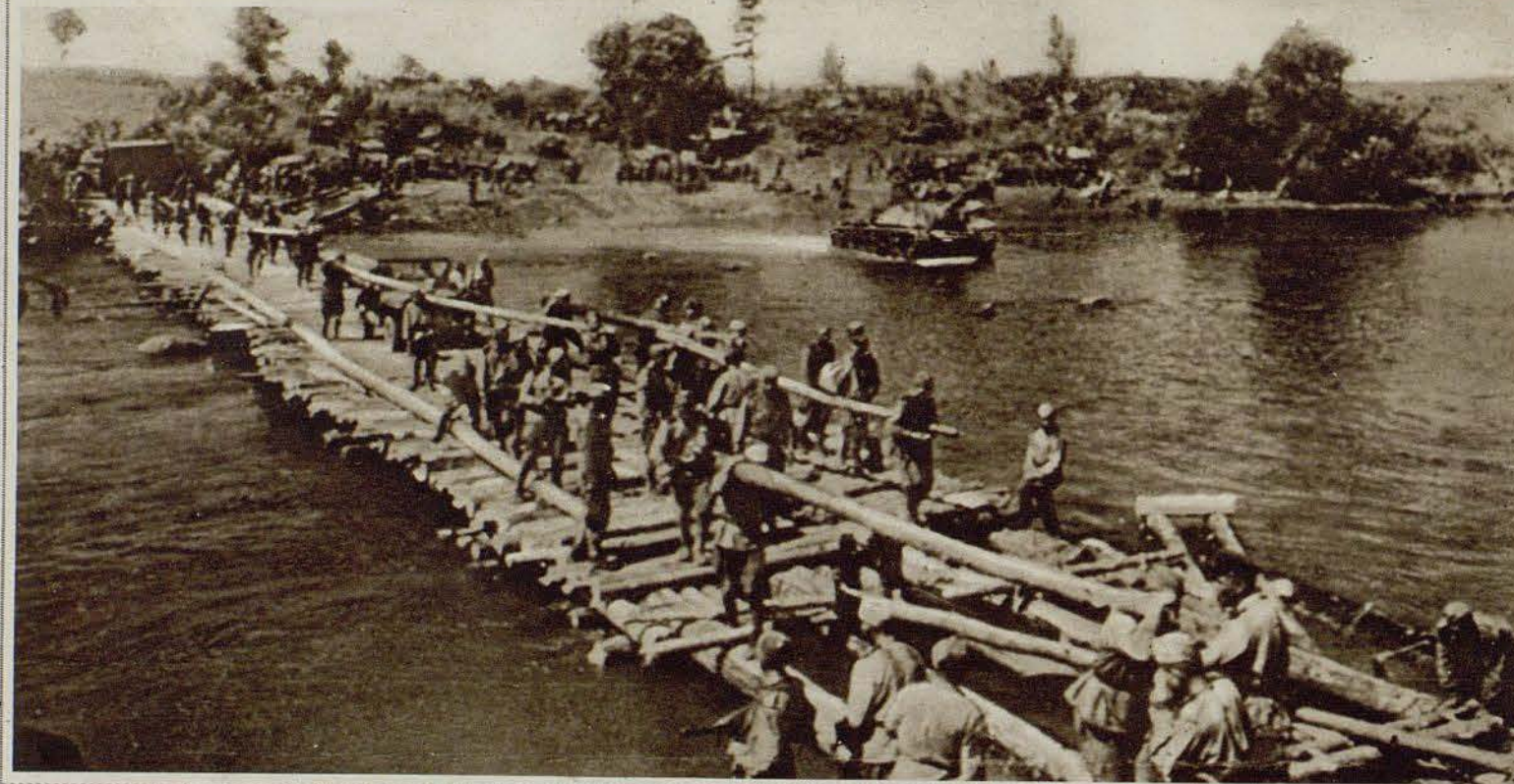
RUSSIAN SAPPERS CONSTRUCTING A BRIDGE FROM TREE-TRUNKS WHILE TROOPS AND ARMOUR WAIT ON THE RIVER BANK IN READINESS TO CROSS. THIS PHOTOGRAPH COMES FROM THE SECOND BALTIC FRONT.
