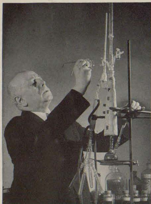
DR. BERL INSPECTS STILL WHICH CRACKS CRUDE OIL
