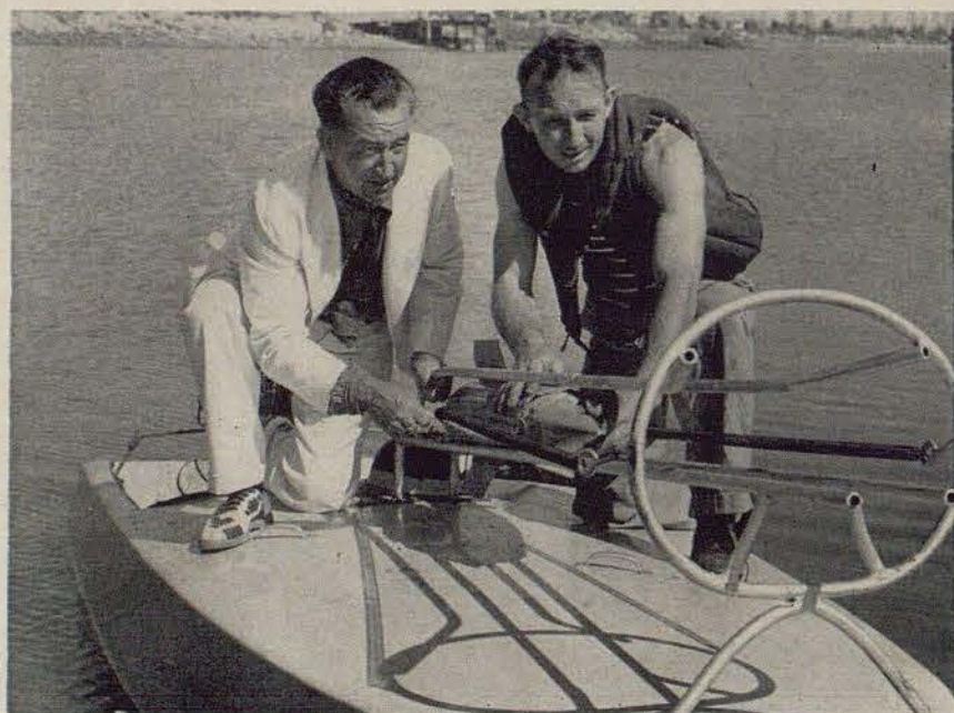
Torpedo tube , to be mounted on outboard motorboats, is demonstrated by Harry Bateson and Smitty Collins. Baby torpedo, launched by springs, would have suicidally short range.
