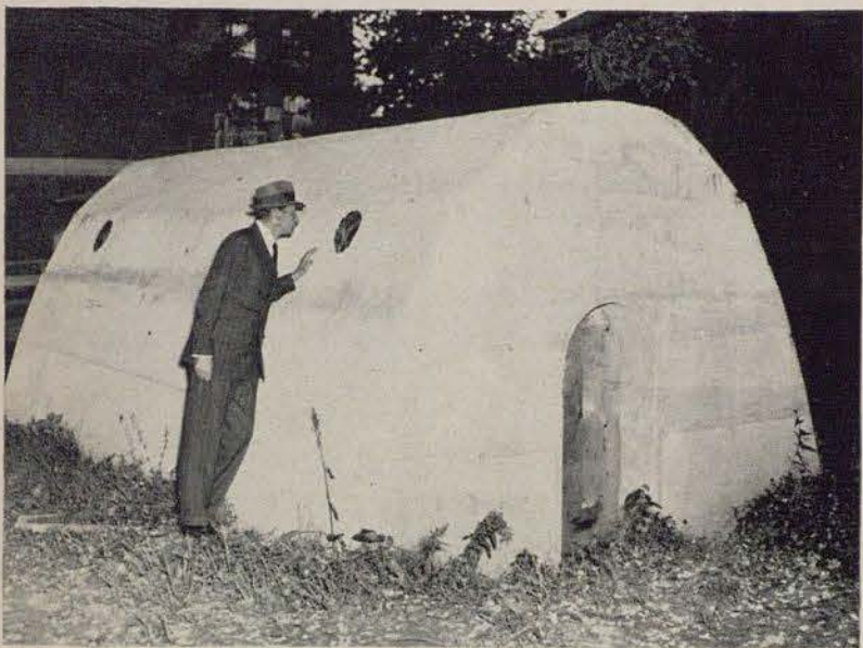
Concrete air-raid shelter was built for tests by the U. S. Bureau of Standards. U. S. Housing Authority is considering plan to add shelters to regular housing projects.
