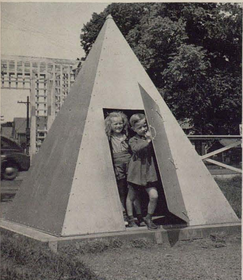
Family shelter was designed by Springfield, Mass. firm on model of popular-priced British shelters. Made of quarter-inch steel, it is not designed to resist direct hits.
