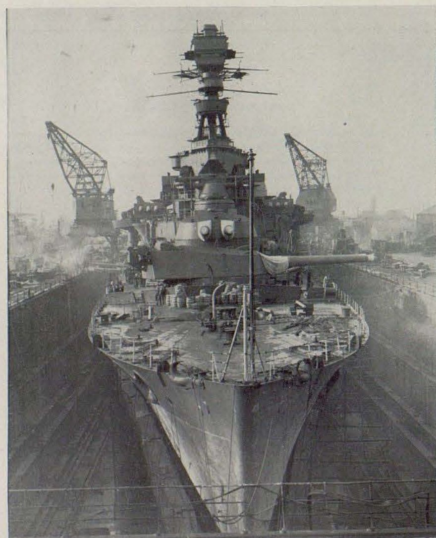
In Portsmouth drydock before the war, the 32,000-ton Repulse gets a complete refit, heavier armor and new 15-inch gun linings. Germany claims to have sunk her, without any proof.
