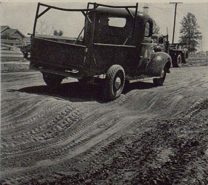
The main road to the main pool has been chewed into deep ruts under constant use by heavy trucks and tractors. It is scheduled for concrete-surfacing in near future.
