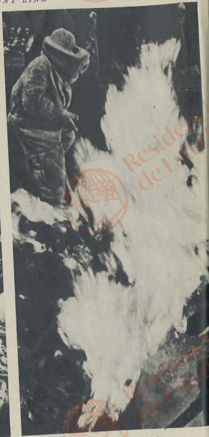
FLAMING GAS. Severed mains break into sheets of fire. They are targets for the enemy and must be plugged while the bombs fall.
