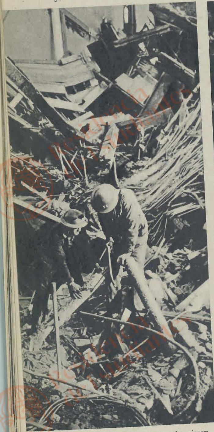
TORN CABLES. Steel-helmeted engineers dig deep into the rubble to repair the cables which carry the city's light and power.
