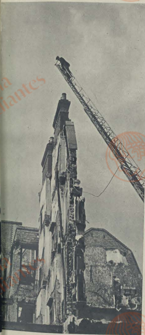
DANGEROUS RUINS. Unsafe walls must be pulled down—the demolition man attaches a steel hawser.
