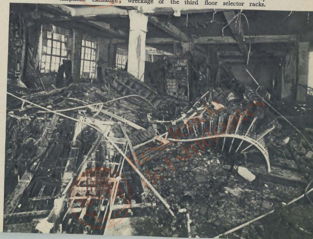
SHATTERED COMMUNICATIONS. A direct hit on a City telephone exchange; wreckage of the third floor selector racks.
