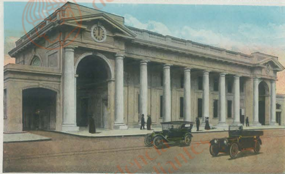
VIEW OF NEW PASSENGER STATION, PANAMA CITY.
