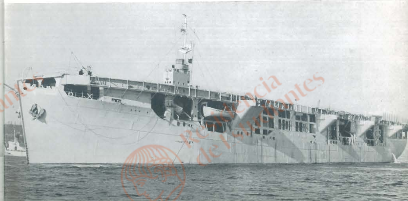
DOWN CAME THE BRIDGE, the funnel. When she was flat, they laid a flight deck on her.
