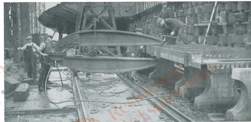
THE LOBSTER CLAWS of the hydraulic riveter, a machine used on prefabricated work
