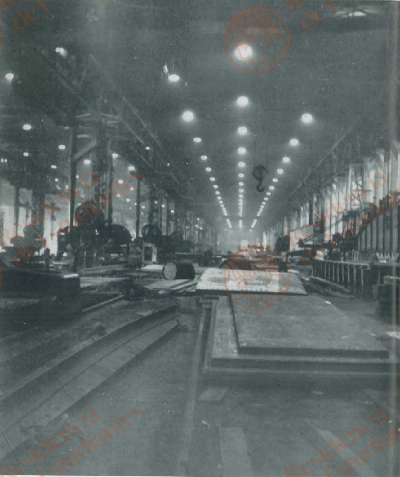
"LIKE SOME PROFANE CATHEDRAL, dim, solemn and portentous," is the platers' shed, where the platers' squad and the frame-benders shape out in metal the template designs for the ship's hull.
