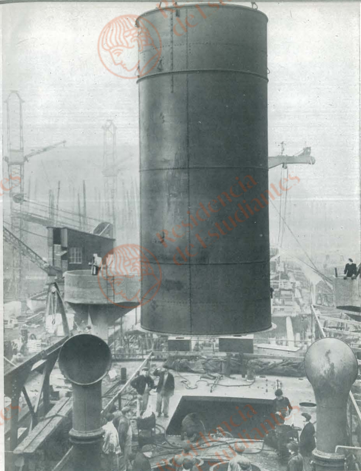
SLOWLY THE GREAT FUNNEL swings into place; the huge, stork-line crane handles it with ease. Below, the riveters wait.
