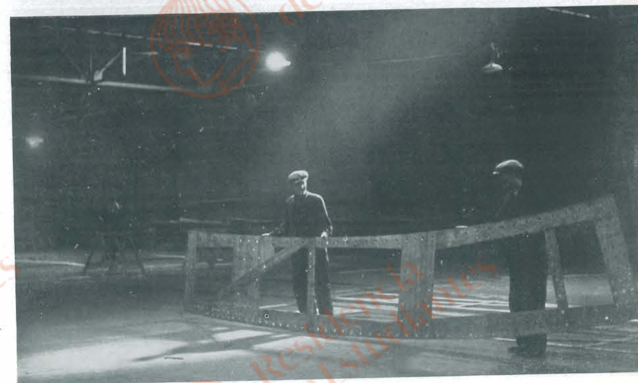
HOW IT BEGINS. In the drawing-office, a high, light, silent room, plans and models are prepared. Templates, full-scale wooden patterns of the ship's plates and frames, are then fashioned in the mould loft.
