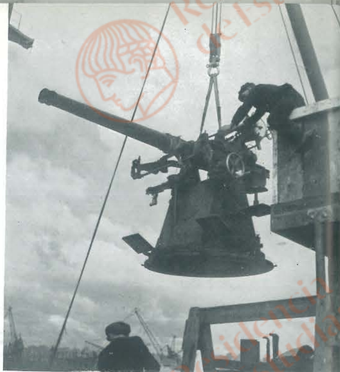
IN A LAST-MINUTE HUSTLE, while the new ship lies at the fitting-out wharf, guns are hoisted aboard, welders flicker over the gun platforms. She is almost ready.
