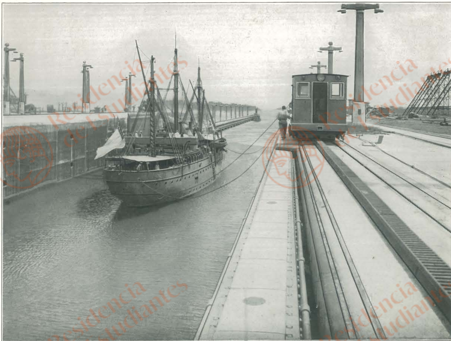
Submarine Tender "Severn" being towed through Gatun Locks by Electric Locomotive (Mule) Panama Canal. Remolcador de Submarinos "Severn" remolcado por Hilanderas Electricas en las esclusas de Gatun, Canal de Panama.
