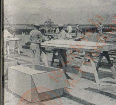
Preparing special bats of Red Top Insulating Wool for installation in plants
