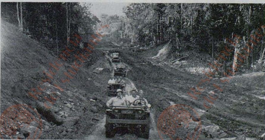
In Panama, the first U.S. Army jeeps try the new Trans-Isthmian Highway, emergency road carved through heavy jungle and hills, now getting all-weather paving.
