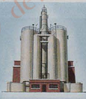
TO PURIFY GAS. The Koppers Seaboard Gas-Purification Process is widely used for the treatment of natural, coal, refinery and water gas.
