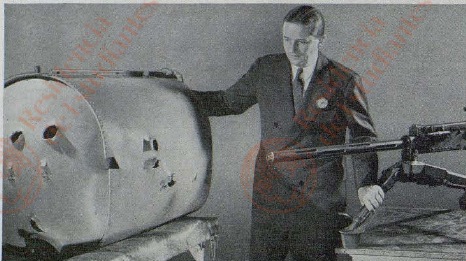
STANDING BETWEEN A 50 CALIBRE MACHINE GUN and one of his aviation gas tanks, Tom Robins, president of Hewitt Rubber Corporation, shows the terrific punishment these tanks must withstand. Hewitt is one of the largest producers of self-sealing gas tanks for fighting planes, and the first to go into big scale production.
