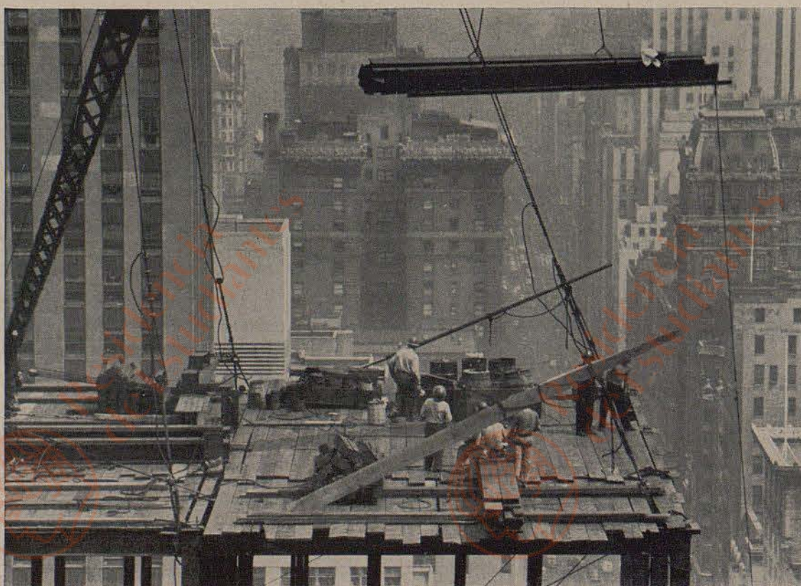
LAST LOAD of beams and girders hovers above workmen as it is swung up out of street and lowered
