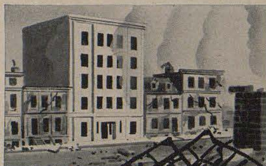
BUILDINGS ARE DAMAGED within mile of the burst. Plaster is cracked, glass is shattered and window frames and doors are blown in by the blast.
