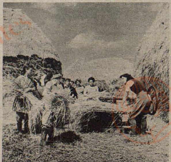
THE GIRLS ARE SHOWN by Miss Burgess how to make a thatch on a haystack. They learn to prepare these thatched roofs which are essential for the protection of the stack against the weather and dampness which, paradoxically, sometimes causes them to catch fire
