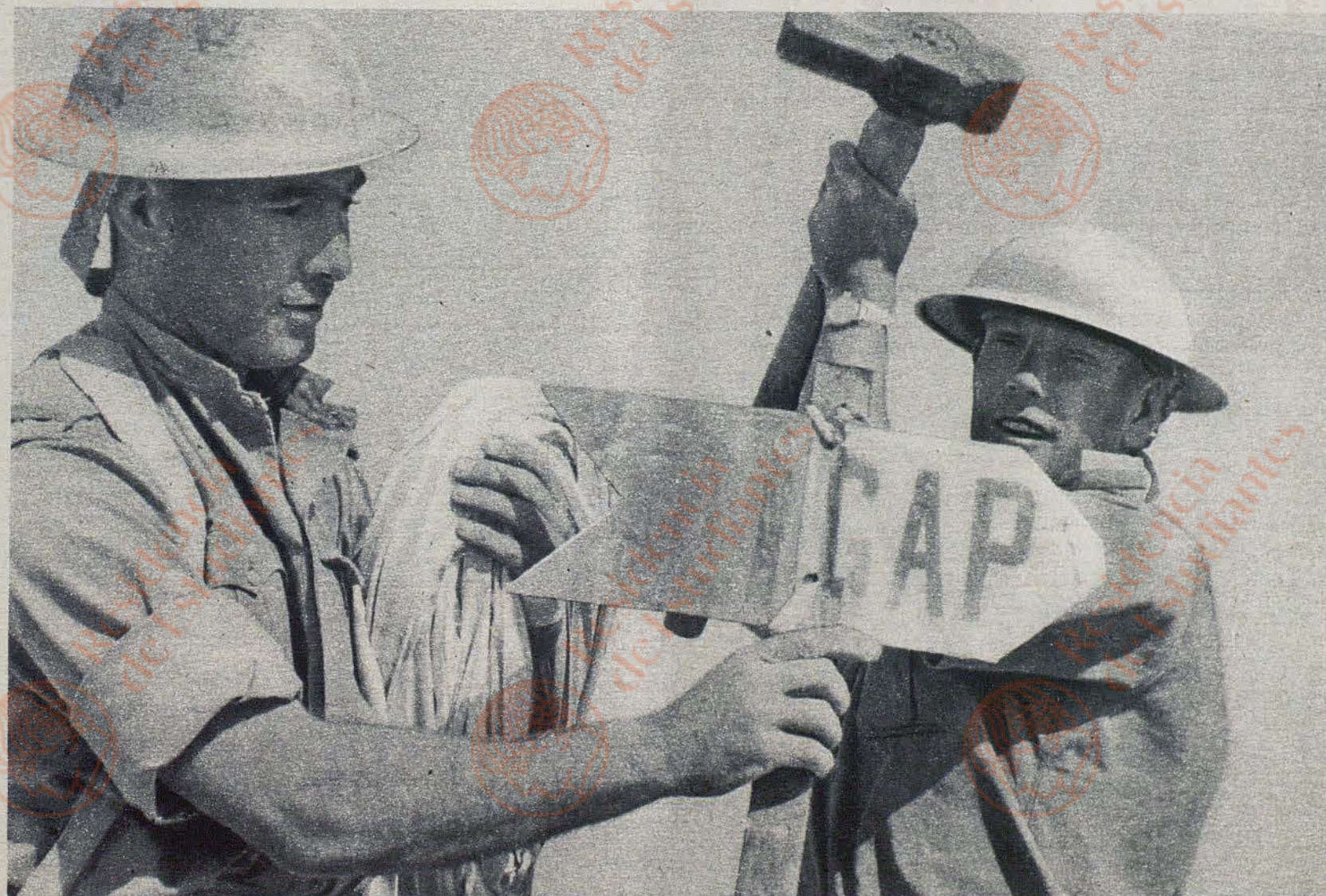
THE GAP IS CLEAR FOR THE TANKS. THE SIGNPOST IS HAMMERED IN, WHITE POINT TOWARDS THE GAP, RED TAIL TOWARDS THE UNCLEARED FIELD.
