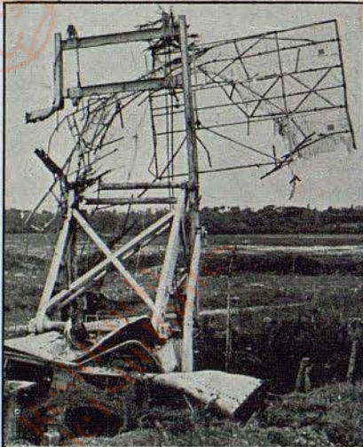
Coastwatcher Radar: This small set was used to detect approaching surface vessels. It was completely destroyed.
