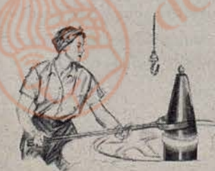
Pressing rotating bands on shell
