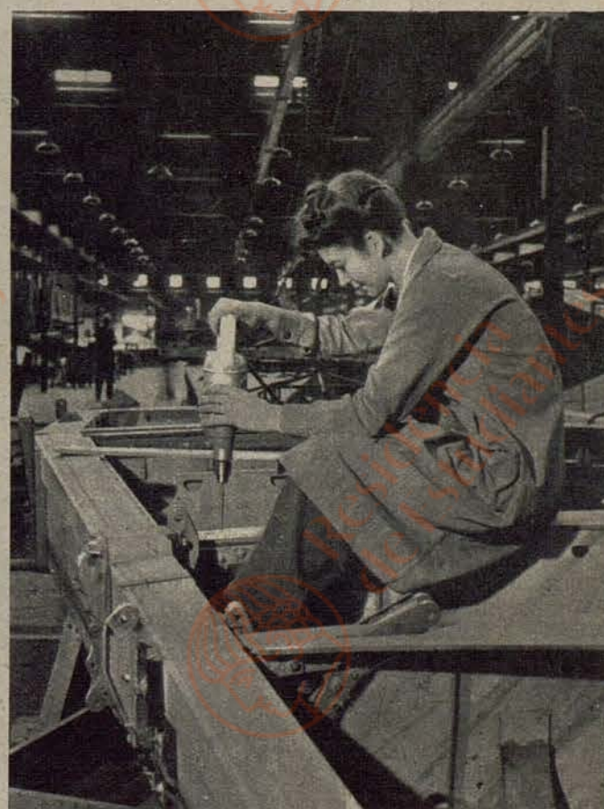
10 The Last Holes are Drilled Women quickly learn to work in the simple jigs which hold the components in position.
