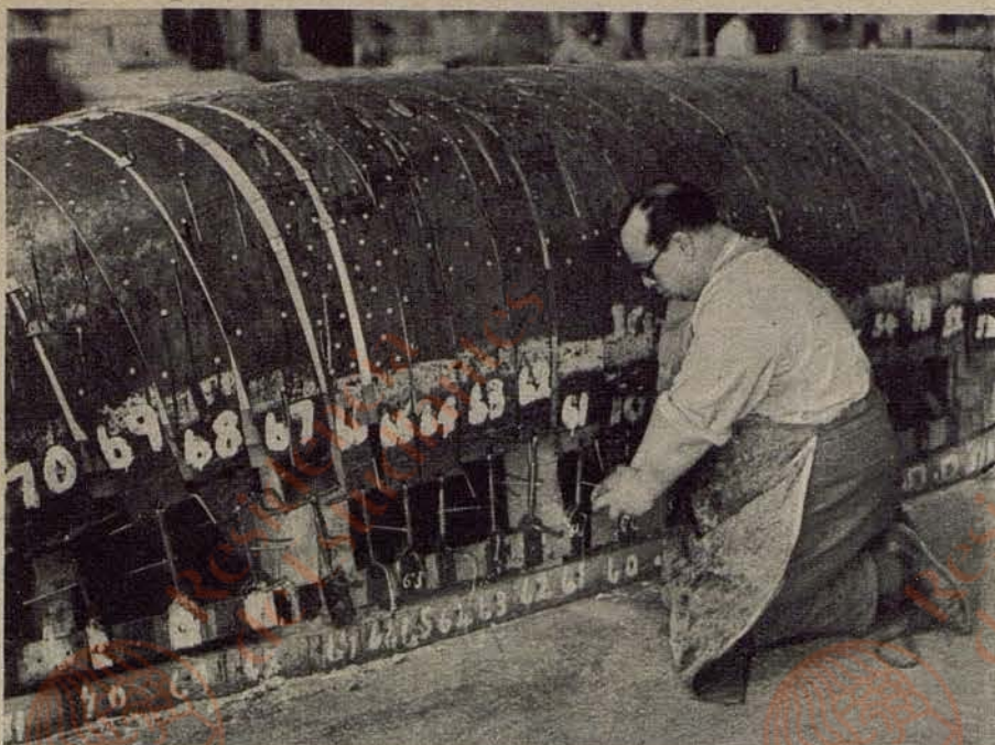
13 The Outer Skin is Strapped Down to Adhere to the Balsa Thin strips of metal clamp the plywood on to the balsa filling. It is left in this position for some hours while the sandwich sets.
