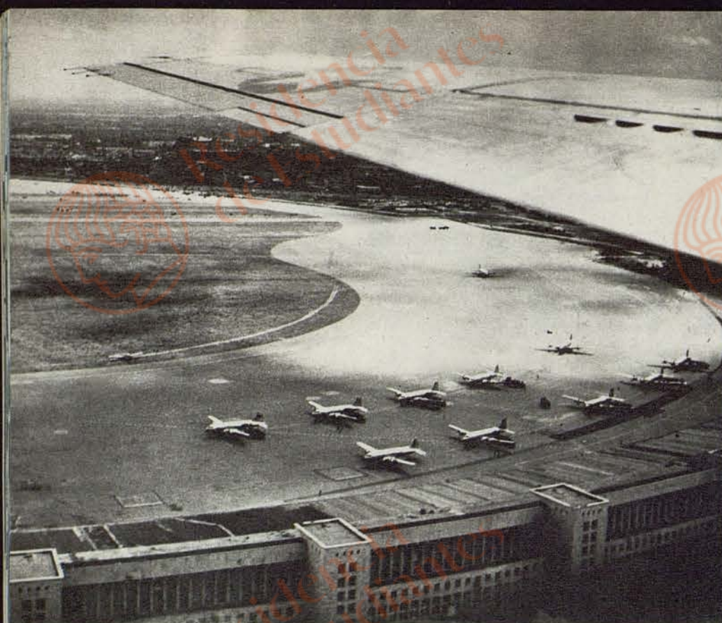
TEMPELHOF, Berlin's capacious pre-war airport, was a ready-made terminal for the Americans. Near the city's centre, it was convenient for dispersal of supplies. But even at Tempelhof the one runway proved inadequate, and two more had to be built.
