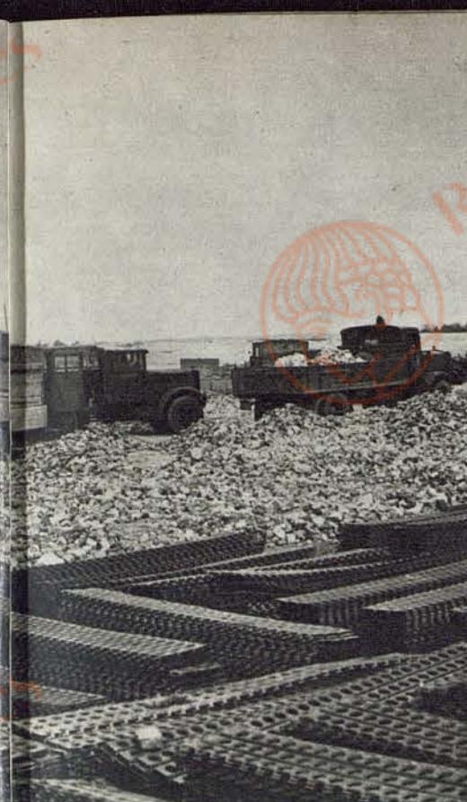
were laid down and a pipe-line for discharging oil-fuel into barges. In the foreground above, pierced steel planking for one of the runways.
