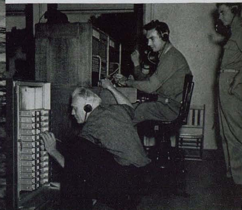
Small military posts as well as big ones need more telephone service. Here a Western Electric installer completes a P.B.X. job for an Army office near Utica, N. Y.
