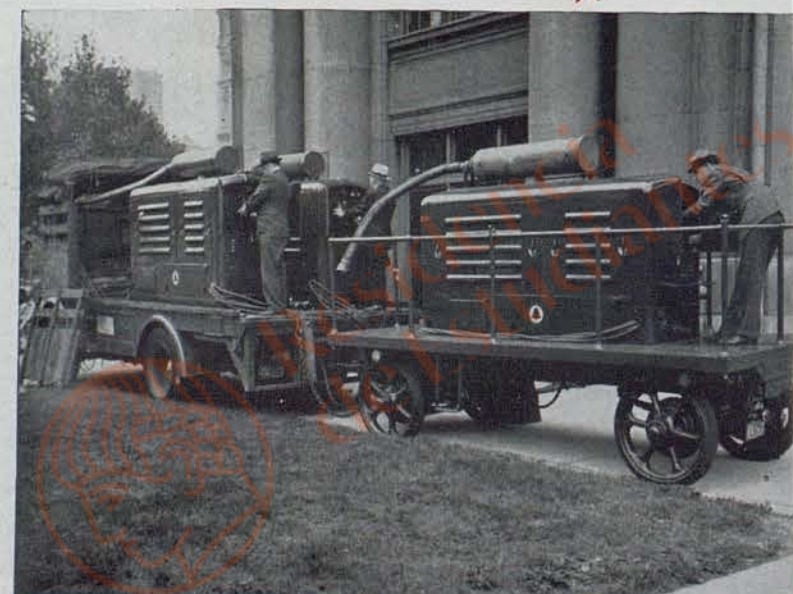
Portable generators help assure continuous power in emergencies.
