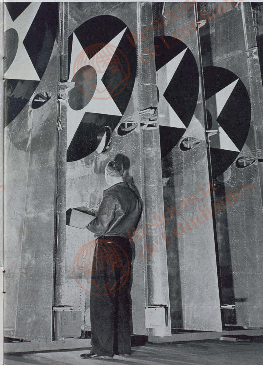
Checking completed wing panels in Boeing plant before final assembly.
