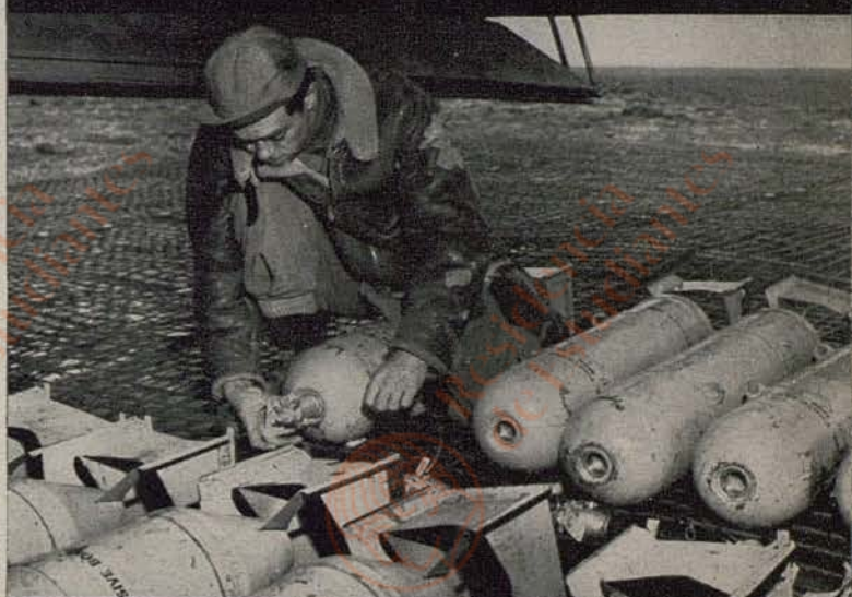
An ordnance mechanic sets fuzes of the flash bombs which, upon explosion, will emit light equal to 800,000,000 candlepower.
