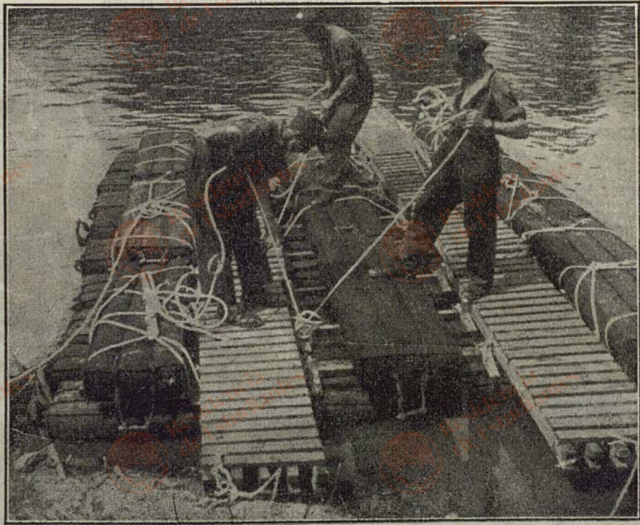
FIG 33.—Improvised raft for 15-cwt truck
