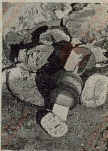
FIG. 25.—DEMOLITION SET PLACED READY TO BLOW A No. 68 "BLIND"
