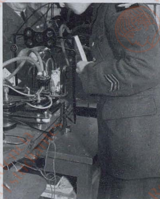
Assembling the "Gyro-Pilot," the machine which can take over control from the pilot for short periods on a flat course.
