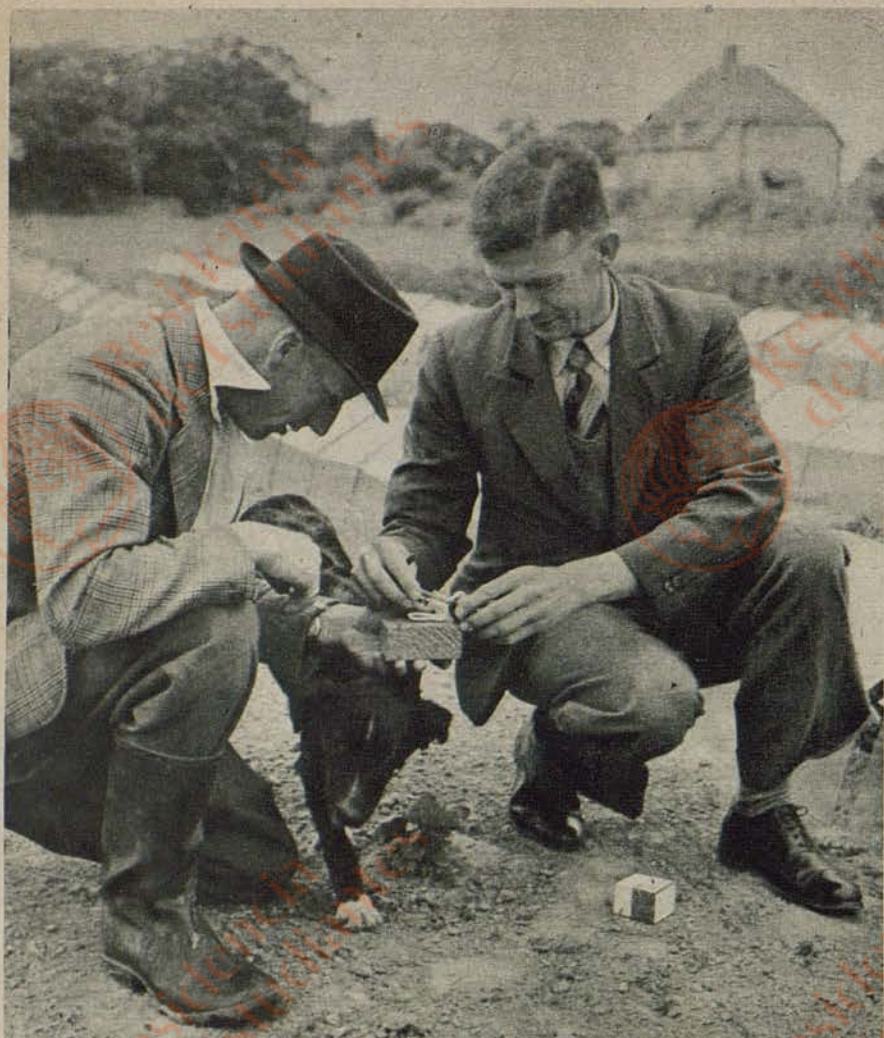
Soil Tests are provided for tenants under the Land Settlement Association. Mr. Edmond Knight is seen testing soil from Mr. Jeffrey Godden's holding for lime content
