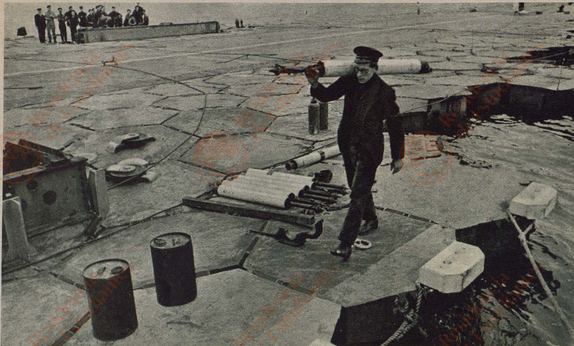
ONE OF THE GROUND CREW BRINGS UP ROCKETS TO ASSIST THE PILOT IN THE TAKE-OFF. THIS CLOSE-UP VIEW GIVES SOME IDEA OF THE SIZE AND CONSTRUCTION OF THE LILY AIRSTRIP
