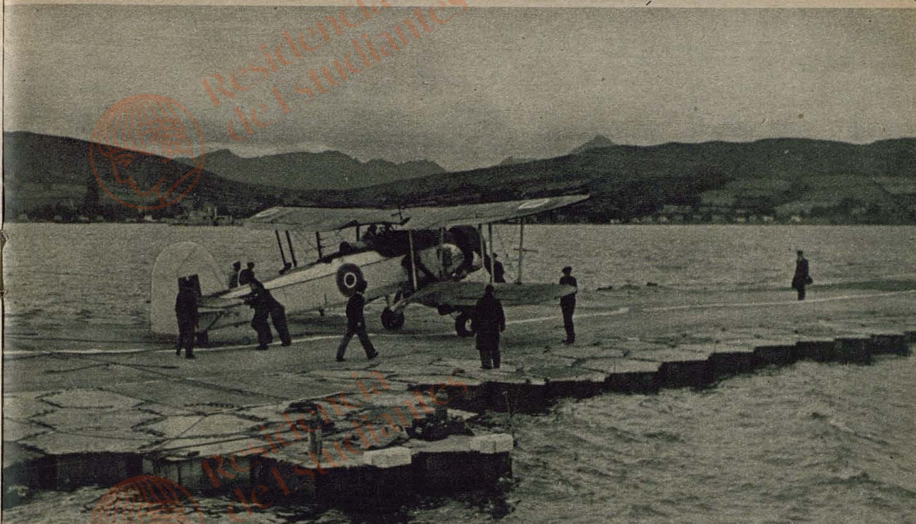
BREAKABLE RUNWAY ON THE SURFACE OF THE SEA. NOTE HOW THE WEIGHT OF THE PLANE BENDS THE SURFACE OF THE AIRSTRIP, AS THE IRON WEIGHT BENT THE MODEL IN THE BATH
