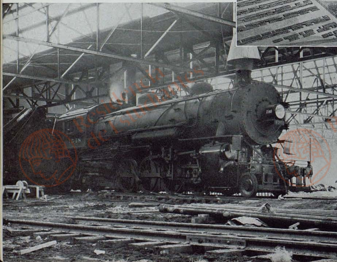
TWENTY MILLION POUNDS of structural steel is being riveted into place at the Cincinnati plant by steel workers such as these. In order to move this structural steel into the plant more than a mile of temporary railroad track was built inside the factory.
