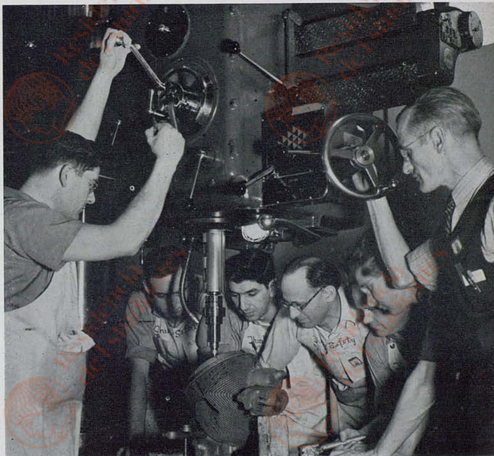
THESE TRAINEES are watching intently as a learner receives instruction on a radial drill, shown here as it drills and reams valve guide holes in a Cyclone cylinder head.
