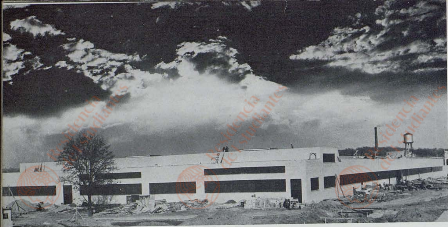
CYLINDER HEADS will be produced in the 161,000 square foot aluminum foundry of the Cincinnati division shown above. The first casting is scheduled to be turned out April 15. Electric hoists, conveyor chains, overhead monorails, electric jaw crushers, motorveyors and chutes have been installed to accelerate manufacture of the heads for Cyclone 14's.
