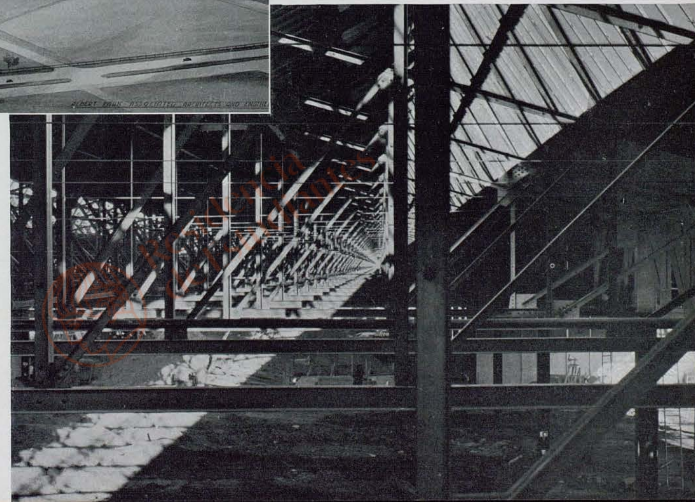
AN IDEA OF THE SIZE of the main building in the Cincinnati plant can be obtained from this photo of the structural steel. In order not to delay production, as each section is completed, plywood is used for inter-section partitions to protect machines and operators from the elements and from construction operations in the adjoining sections.
