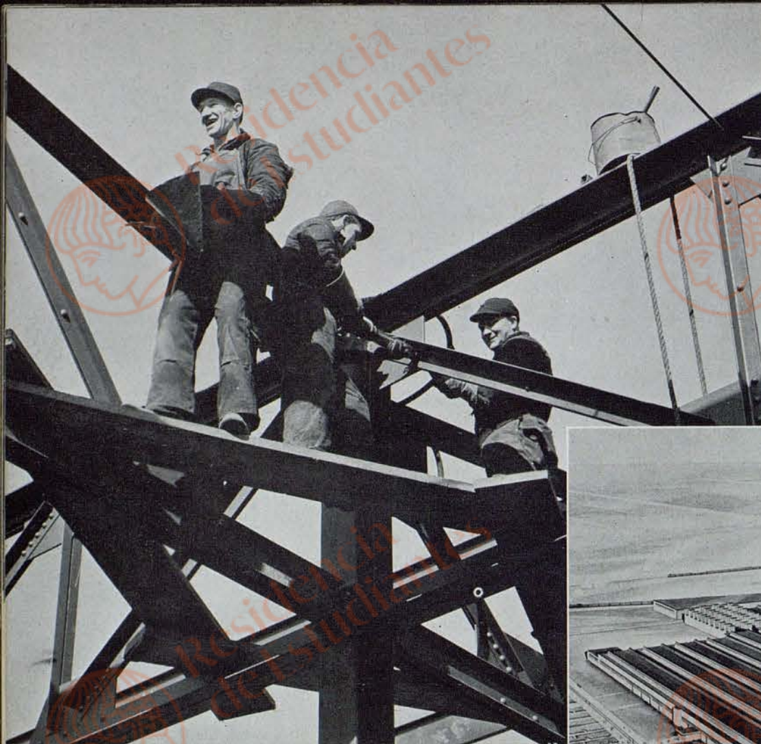
TWENTY MILLION POUNDS of structural steel is being riveted into place at the Cincinnati plant by steel workers such as these. In order to move this structural steel into the plant more than a mile of temporary railroad track was built inside the factory.
