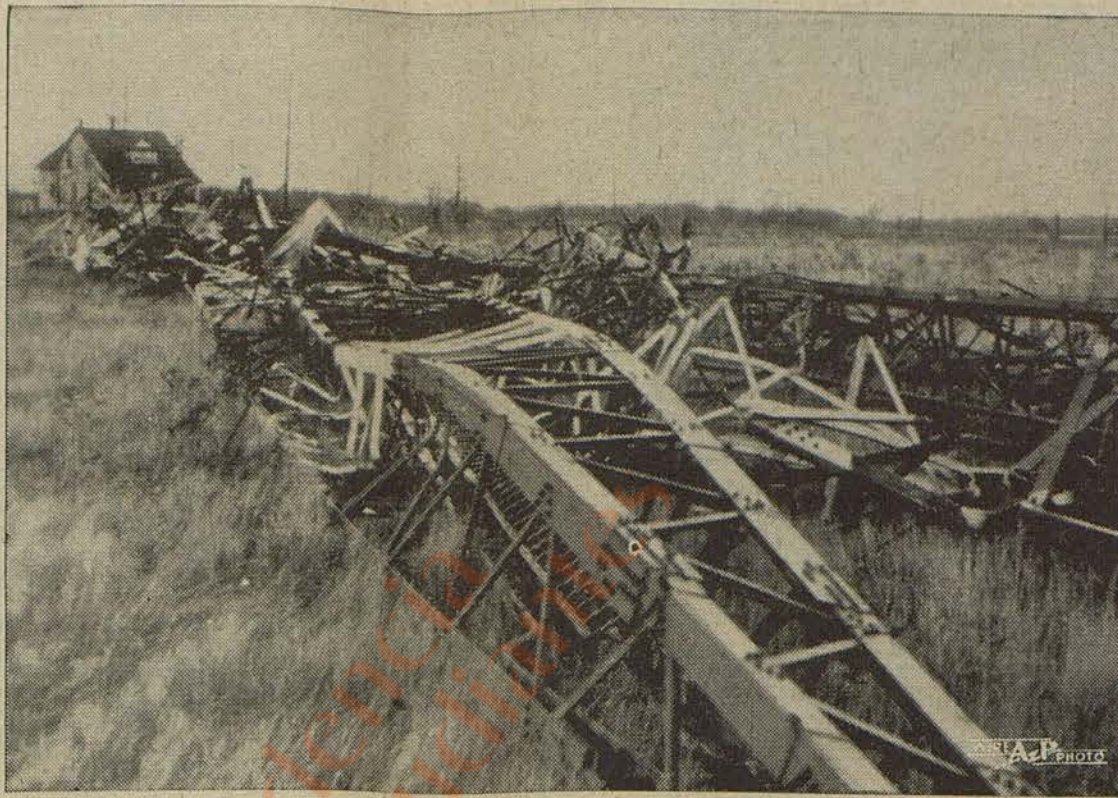
733-foot steel antenna tower of radio station WJR, the tallest structure in Michigan, was toppled by gale winds. Damage to the tower was estimated at $60,000.
