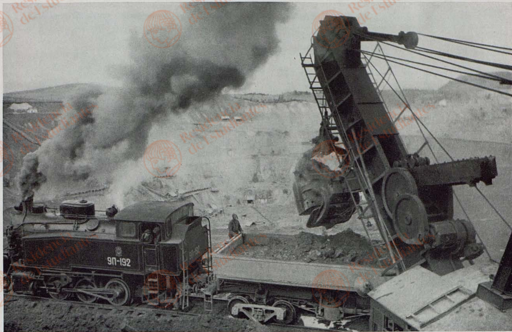
An Electric Excavator Dumps a Mighty Mouthful of High-grade Iron Ore into a Car at an Open Pit in the Urals
