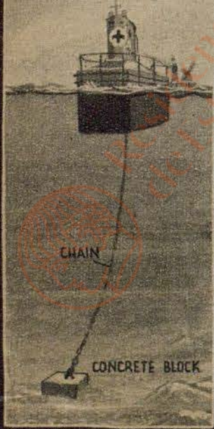
METHOD OF MOORING BUOY TO SEA-BED
