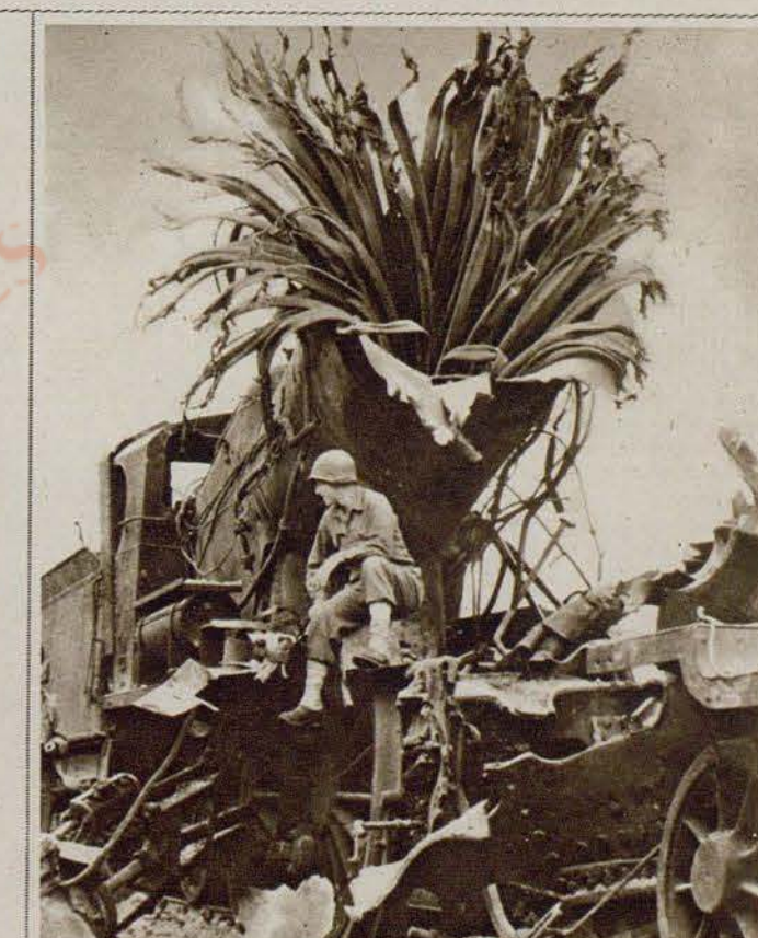
NOT SOME EXOTIC PLANT, BUT THE INTERNAL TUBES OF A LOCOMOTIVE, HIT BY ALLIED BOMBERS AND TORN TO SHREDS.
