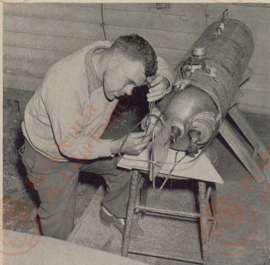
Torpedo-mine , invented by Leslie Crosby of Springfield, Mass., is released and guided to its objective by the sound of a ship. The present war has revealed several new mines in operation.
