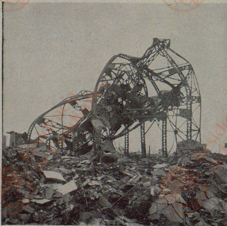
Steel girders of another factory were twisted into knots, while the wall casing shot away and fell to the ground in rubble. Under the full blast, most Hiroshima factories just disintegrated.
