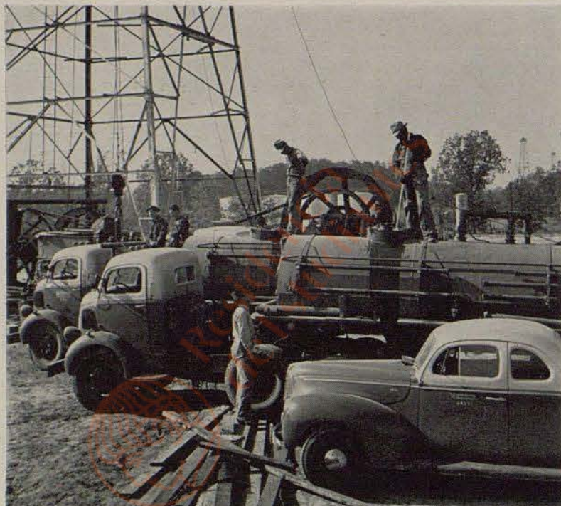
Acid is pumped into a well to eat away deep limestone, open up producing zone. The man on tank truck is using a measuring rod to determine how much acid has gone in.
