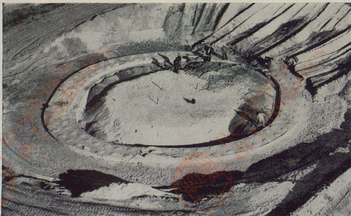
SITE for the cosmotron was excavated in 1949. A concrete base was laid for the machine to rest on, and
